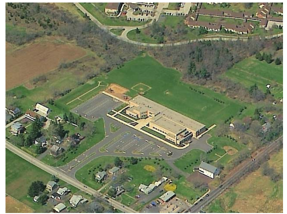
Worcester Elementary School
