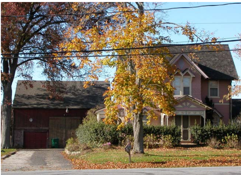
Victorian house on North Wales Road
