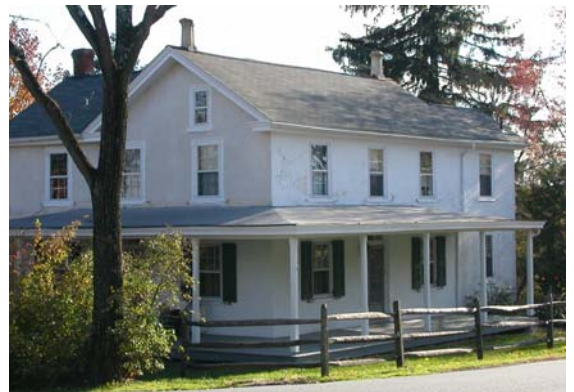
The Lowry / Gouley House at Whitehall and Bean Roads
