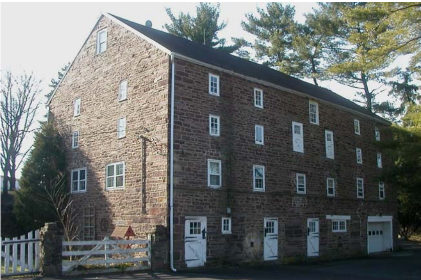
Kriebel Mill barn is along the Zacharias Creek greenway and trail corridor as well as being one of the largest stone barns in the area Photo: Laura Caughlan
