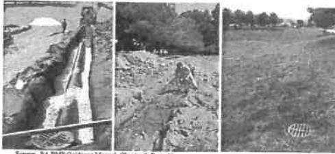
Figure 4: Example of Infiltration Trench Installation
