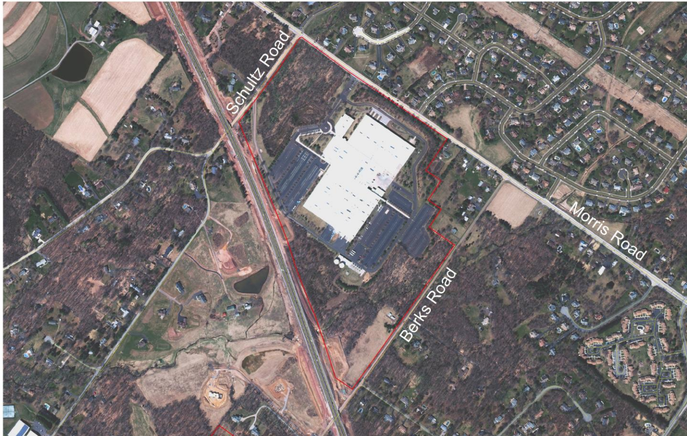
2750 Morris Road - Building "D" South MCPC #19-0007-001
