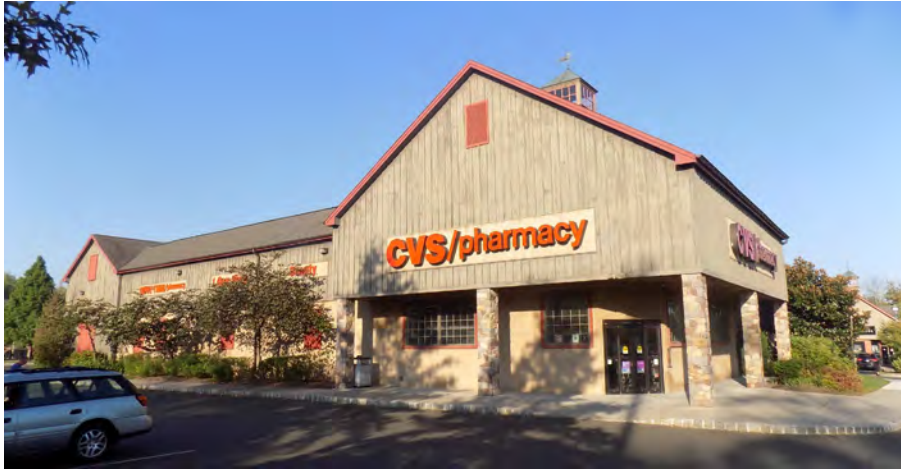
The next two photos are of CVS stores in central Bucks County that attempted to follow traditional styles.
