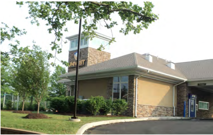
An example of a bank in Doylestown area that uses traditional materials and sets back the drive-through from the street.
