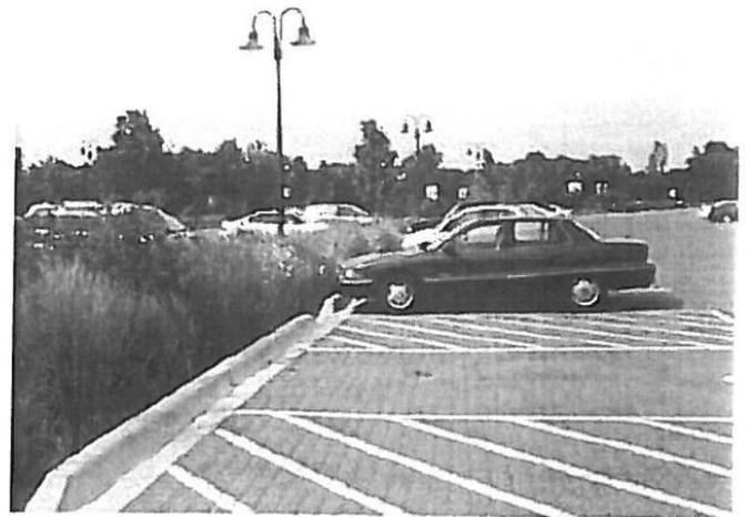
Interlocking concrete pavers work together with curb inlets to provide rainwater to the bioretention area
