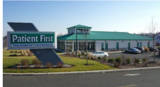
Penn E&R is experienced in site engineering and permitting services for cost-effective land development projects for commercial businesses.
