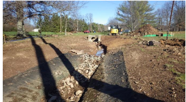
Nearly completed channel restoration.
