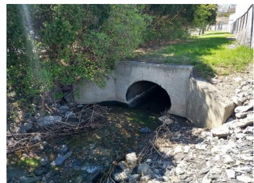
Penn E&R provides permitting and construction services, repairs and maintenance of stormwater control systems.
