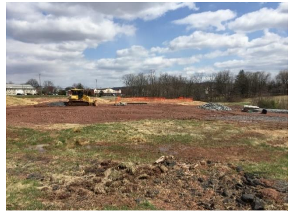
Initiation of site grading at land development site in Eastern Pennsylvania.
